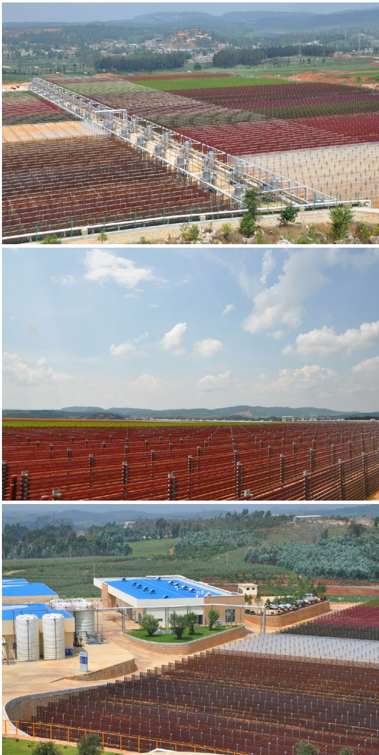
Figure 11. Astaxanthin production plant
